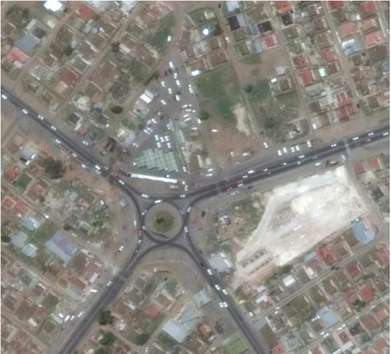
Arial view of project after 72 properties were acquired and demolished
